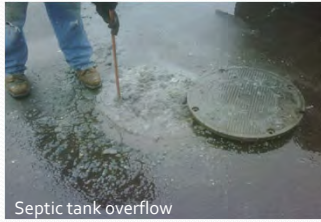
Septic tank overflow
